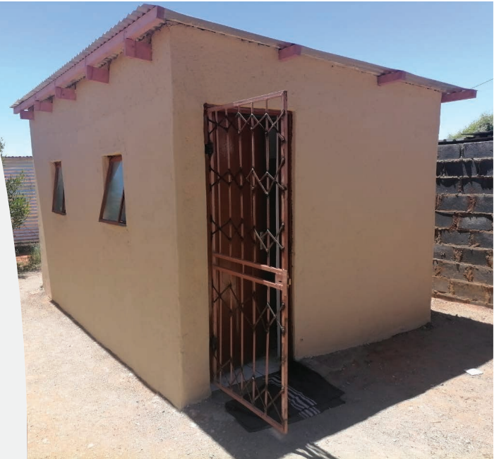
Completed lavatory structure
